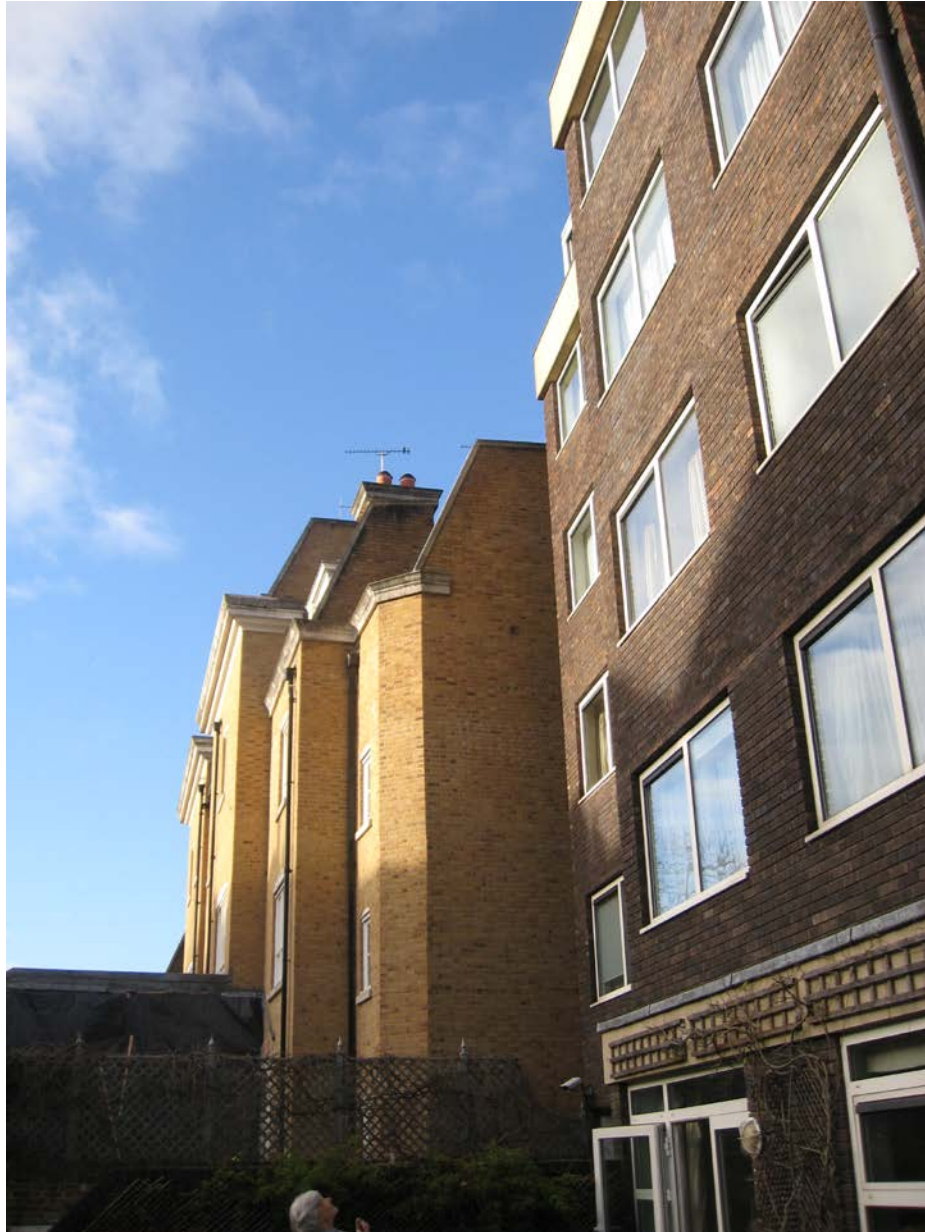
View from the Rear Garden of 45 Marlborough Place
